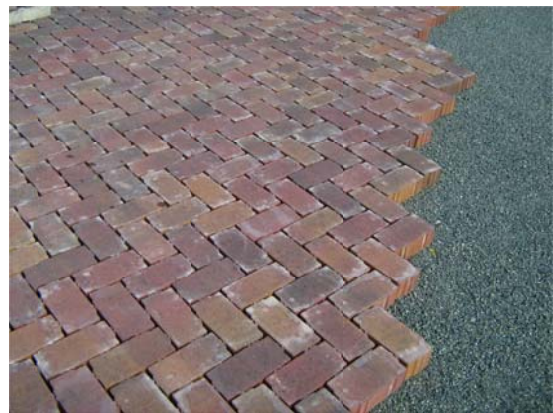
PICP (during construction) at Odell Brewing Co.
