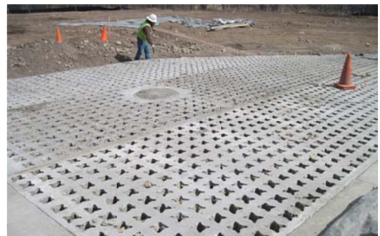
Grasscrete at Mulberry Reclamation Plant (during construction)
