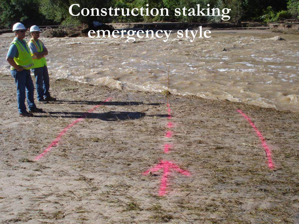
Cutting off an upstream side channel before installing spur #1
