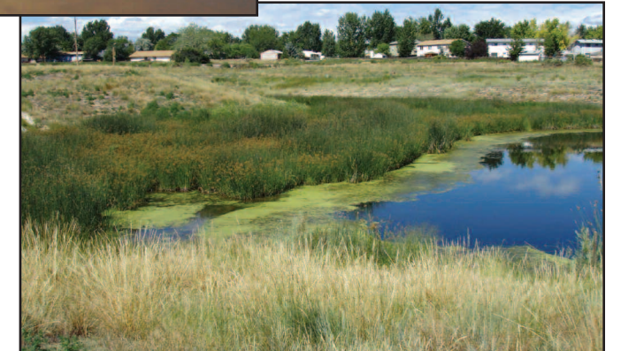
Littoral shelf at southern end of North Pond supports nearly an acre of emergent wetlands in a shallow water habitat. Concrete weir, top, is designed to maintain a 6-inch water depth on the shelf to support wetland plant growth should pond level drop.
