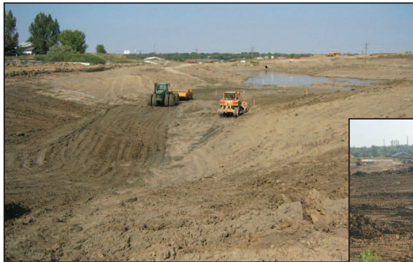
Outlet pipe from north pond is installed, above, as excavation of the site nears completion. With the site dewatered, top right, crews capture normal flows through the site in a temporary pond while muck is excavated for removal by excavators and articulated trucks. Below, grading nears completion on the north pond and its wetland littoral shelf.
