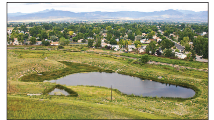
Upland native prairie between the south and north ponds was necessary to allow a safe 4:1 slope or less of the ponds' banks. South, or upper, pond, left, is connected to the north, or lower, pond, right, via a 30-inch concrete pipe, effectively providing temporary detention in the south pond during storm events. South pond is designed to retain about six inches of water.
