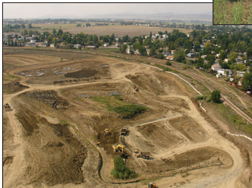
Fort Collins-based Connell Resources Inc. de-watered the site and performed muck removal, grading, material importation and placement, pipeline installation and pond construction.
