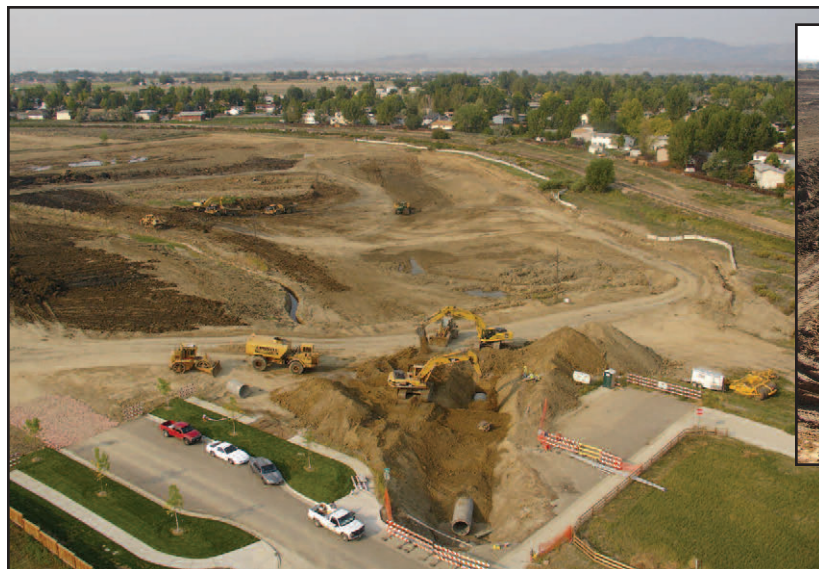
Outlet pipe from north pond is installed, above, as excavation of the site nears completion. With the site dewatered, top right, crews capture normal flows through the site in a temporary pond while muck is excavated for removal by excavators and articulated trucks. Below, grading nears completion on the north pond and its wetland littoral shelf.
