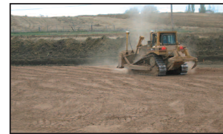
Topsoil was imported and placed for the 1.4-acre shallow water south pond. Sediment basin, below, overflows to water the pond’s wetland vegetation and can be maintained without wetland disturbance.
