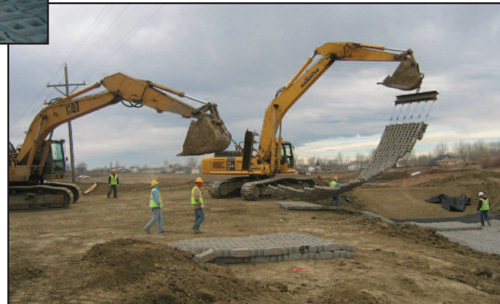
ArmorLoc® concrete interlocking blocks are installed for the inlet of the north pond to effectively control erosion. The system is installed over filter fabric and an prepared subgrade.
