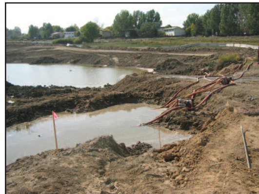
Fort Collins-based Connell Resources Inc. de-watered the site and performed muck removal, grading, material importation and placement, pipeline installation and pond construction.
