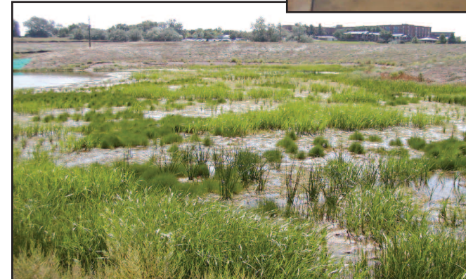
Littoral shelf at southern end of North Pond supports nearly an acre of emergent wetlands in a shallow water habitat. Concrete weir, top, is designed to maintain a 6-inch water depth on the shelf to support wetland plant growth should pond level drop.
