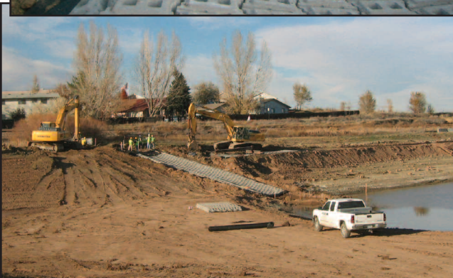
ArmorLoc® concrete interlocking blocks are installed for the inlet of the north pond to effectively control erosion. The system is installed over filter fabric and an prepared subgrade.
