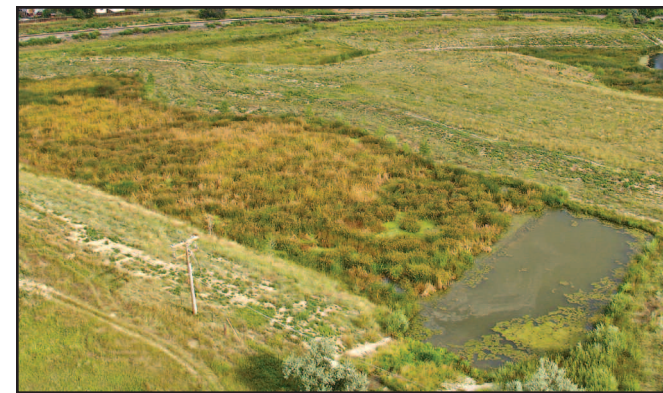
Upland native prairie between the south and north ponds was necessary to allow a safe 4:1 slope or less of the ponds' banks. South, or upper, pond, left, is connected to the north, or lower, pond, right, via a 30-inch concrete pipe, effectively providing temporary detention in the south pond during storm events. South pond is designed to retain about six inches of water.
