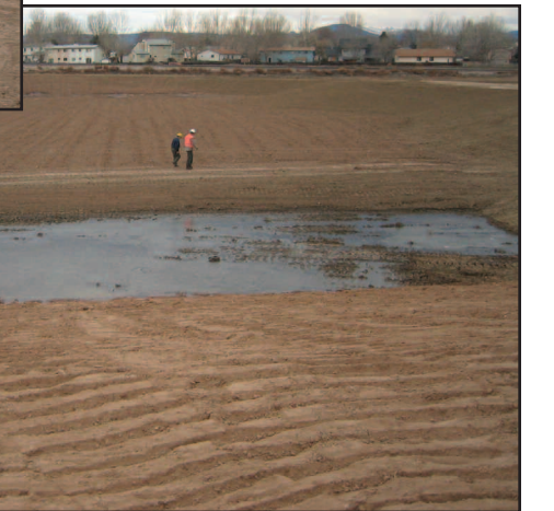
Topsoil was imported and placed for the 1.4-acre shallow water south pond. Sediment basin, below, overflows to water the pond’s wetland vegetation and can be maintained without wetland disturbance.
