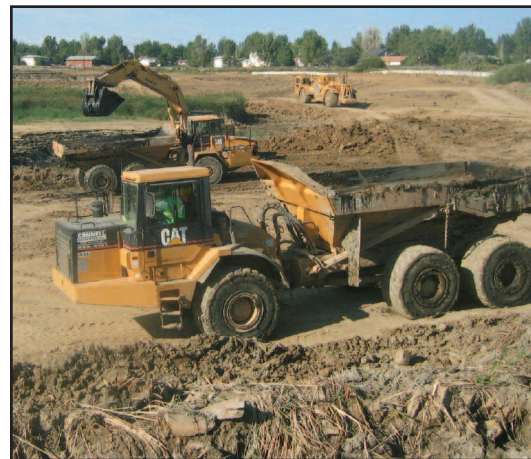
Outlet pipe from north pond is installed, above, as excavation of the site nears completion. With the site dewatered, top right, crews capture normal flows through the site in a temporary pond while muck is excavated for removal by excavators and articulated trucks. Below, grading nears completion on the north pond and its wetland littoral shelf.
