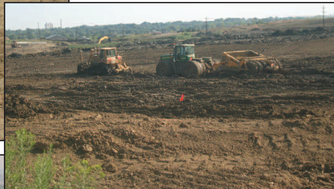
Fort Collins-based Connell Resources Inc. de-watered the site and performed muck removal, grading, material importation and placement, pipeline installation and pond construction.
