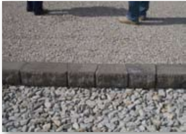
Open-graded aggregate base course layers. Photo by Michelle DeLaria.
