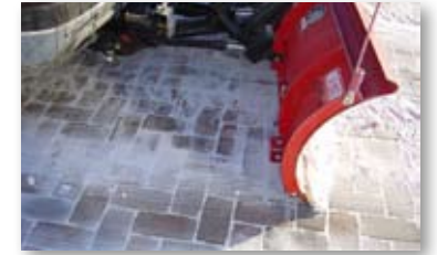
Pavers can be plowed. Photo Courtesy Chuck Taylor (Advanced Pavement Technologies)
