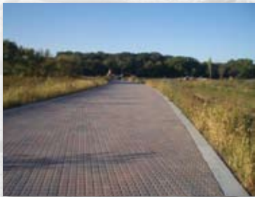
Private road in Illinois with detention capacity underneath pavers. Photo by Michelle DeLaria.
