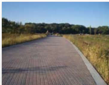
Private road in Illinois with detention capacity underneath pavers. Photo by Michelle DeLaria.
