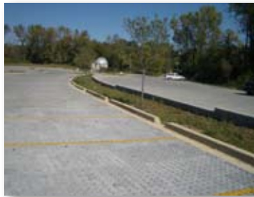
Pavers with the open-graded aggregate system in Illinois and swales for added detention capacity. Photo by Michelle DeLaria.
