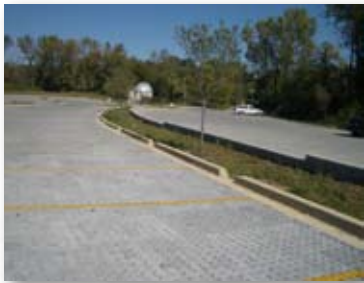
Pavers with the open-graded aggregate system in Illinois and swales for added detention capacity. Photo by Michelle DeLaria.
