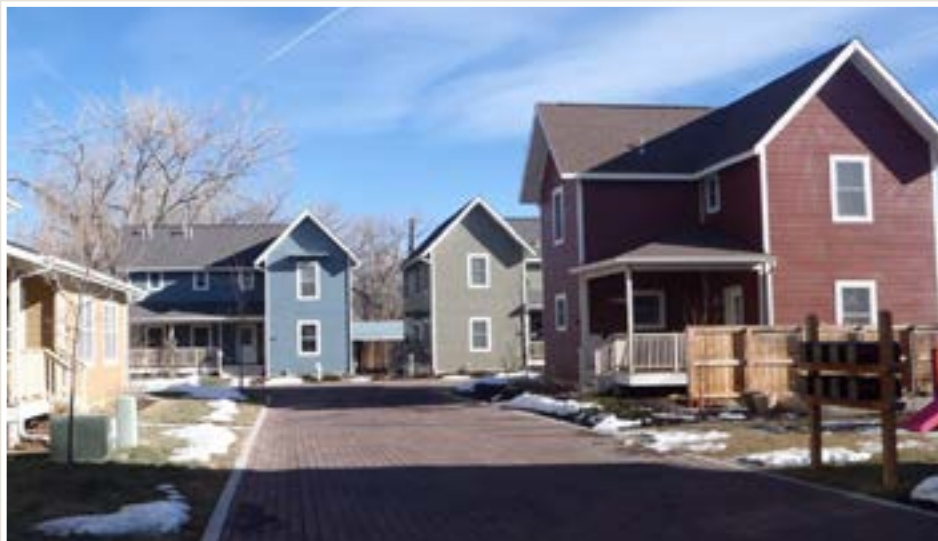
Photo 1. Toby Lane Development in Boulder protected from flood damage in September 2013 because the homes were elevated two feet above the 100-year flood elevation.
