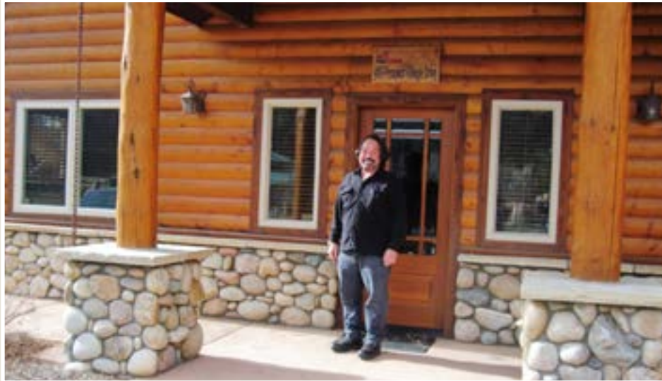
Photo 5. An Estes Park business owner next to his building that was not damaged in the 2013 flooding due to elevating the structure.
