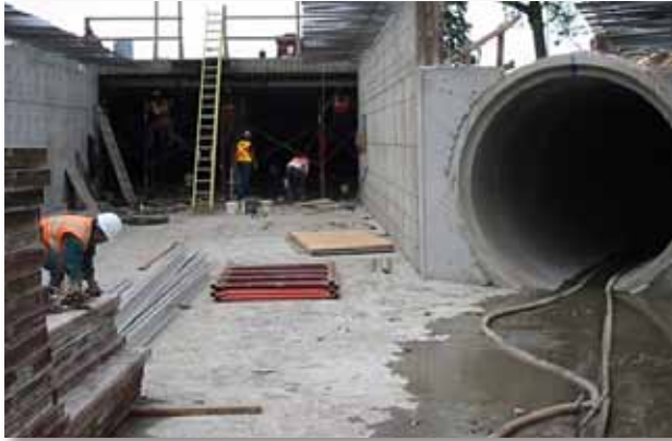
Diversion structure to existing brick storm sewer
