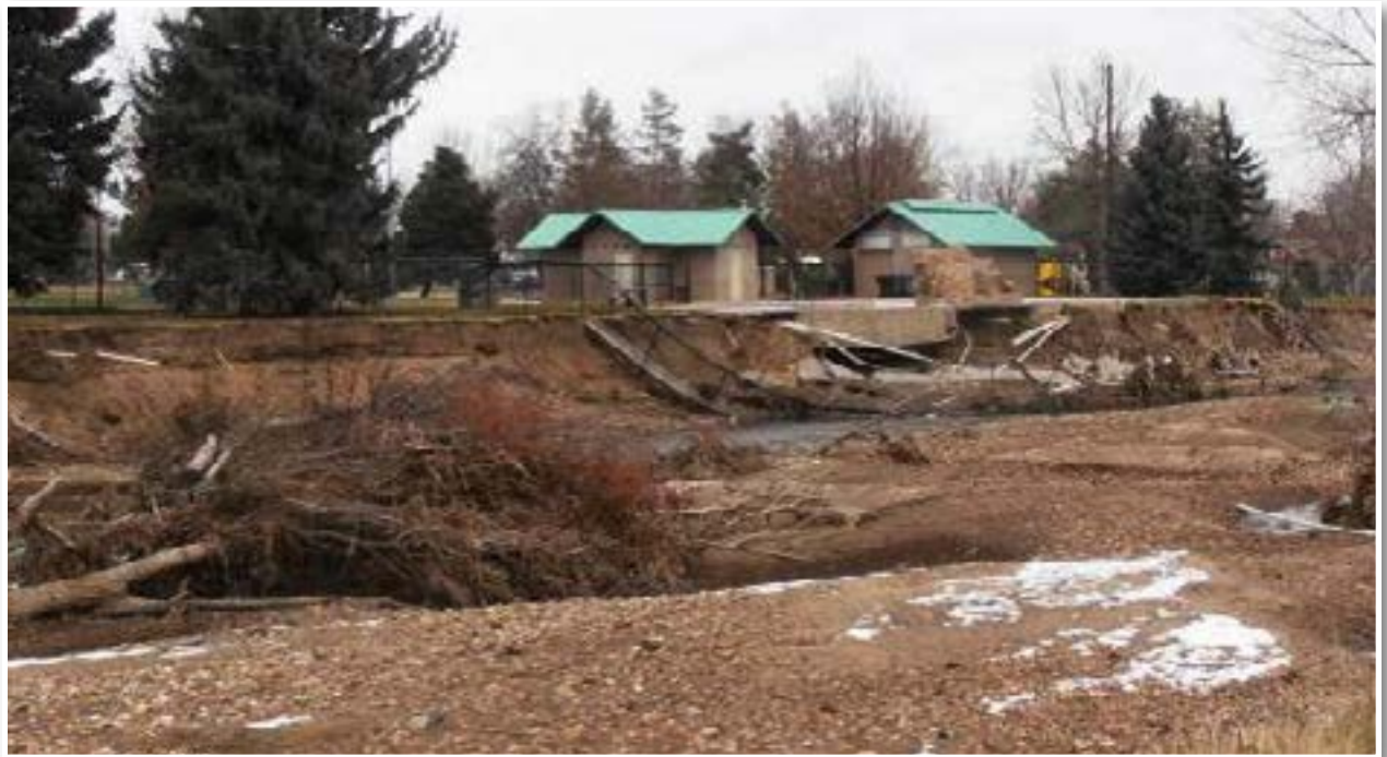
Severe Erosion outside of the Project Improvement Reach
