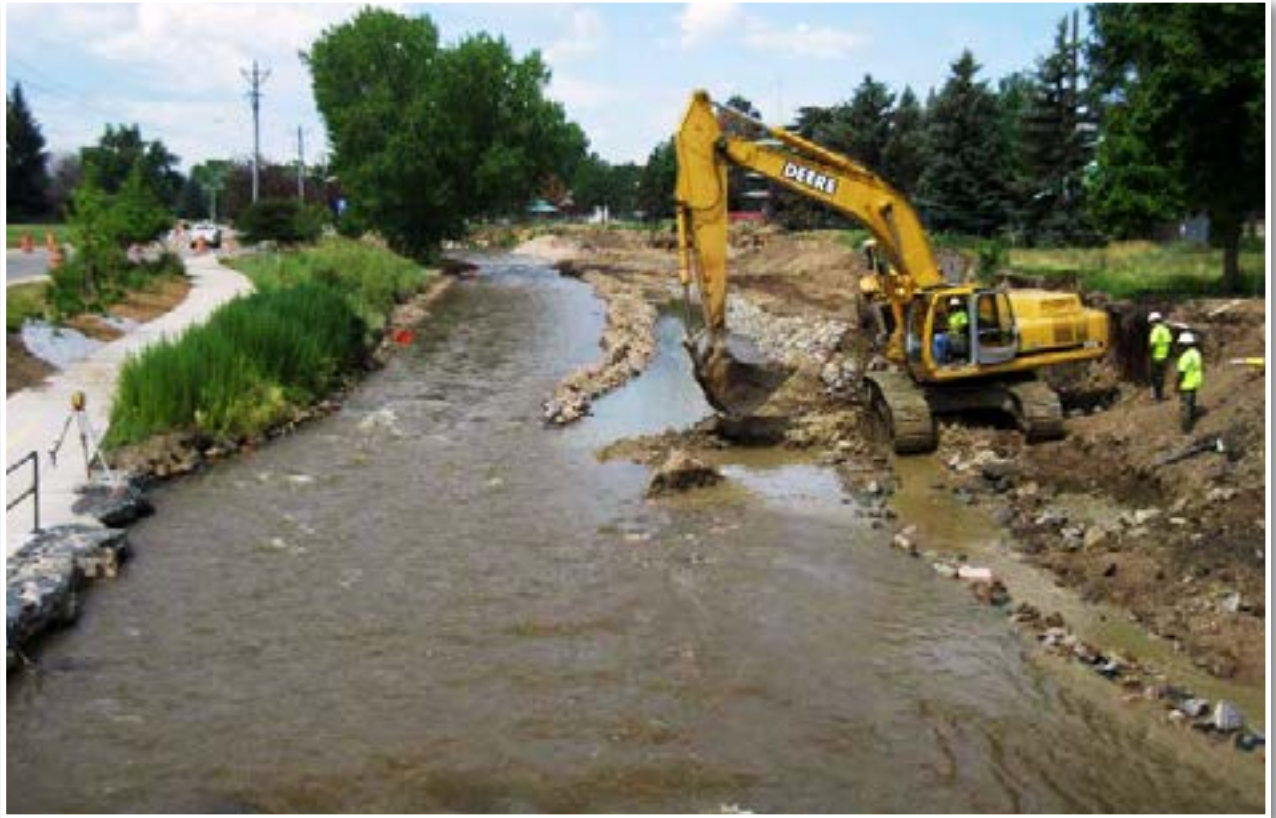
Post Flood Repair Project Underway outside of Project Improvement Reach
