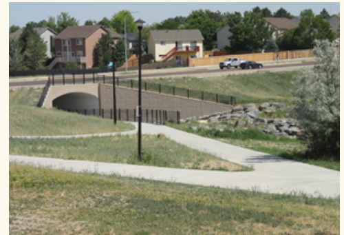
2013 New 100-year capacity crossing structure is 24-ft wide arch with trail underpass. An 8-ft grouted boulder drop structure protects upstream wetlands.
