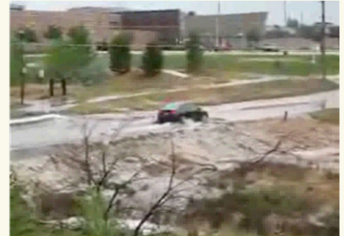
August 6, 2008 (School Registration Day) Holly Street washed out by minor storm event overtopping dual 48-inch CMPs
