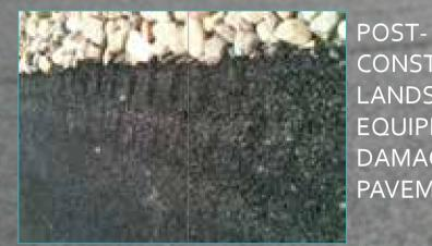
POST-CONSTRUCTION LANDSCAPING EQUIPMENT IS DAMAGING THE PAVEMENT
