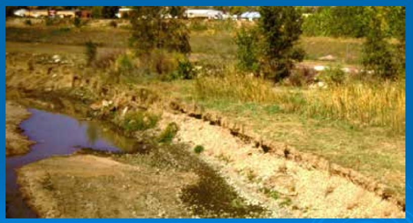
$Q_{design} = 300 \text{ cfs}$   $V_{design} = 4.3 \text{ fps}$  $Q_{100} = 5200 \text{ cfs}$   $V_{100} = 7.2 \text{ fps}$
