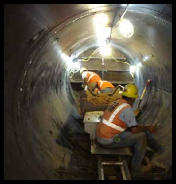
• Tunneling = Construction of a tunnel without disturbance of the ground surface. Also, excavation method relies on manned entry
