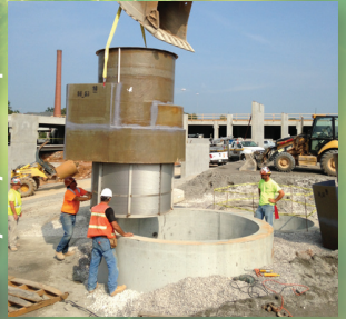
CDS® Hydrodynamic Separator
