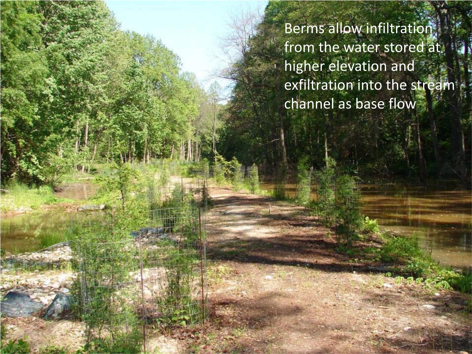
Berms allow infiltration from the water stored at higher elevation and exfiltration into the stream channel as base flow
