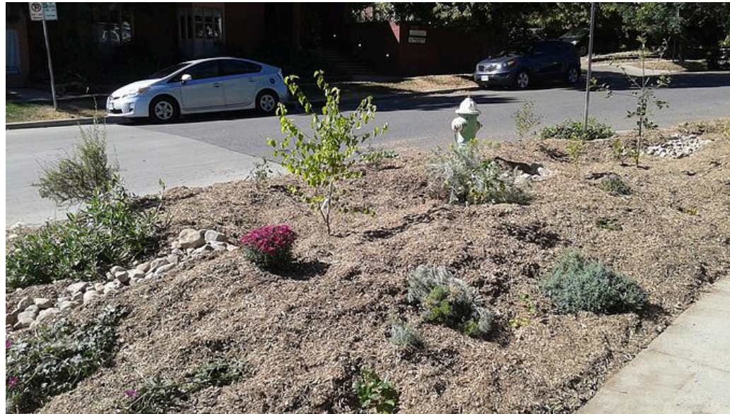
Storm Water Overflow Apron
