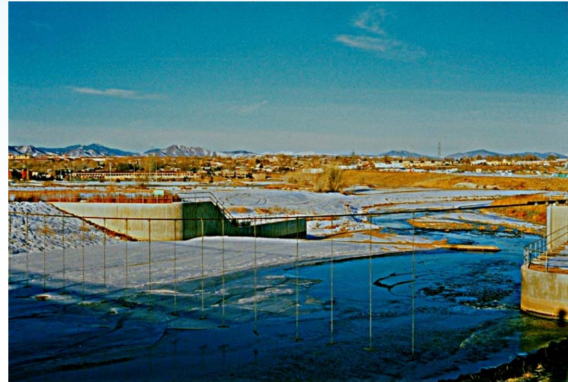
Union Avenue Dam Selected "milder" sloped proved hazardous
